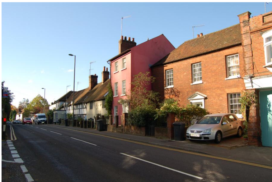
Figure 12: ChA 1 has a variety of architectural styles, but is predominantly 2 storeys with the exception of 78 and 120 Ockford Road
