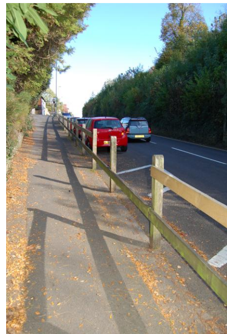
Figure 21: Fencing on Ockford Road
