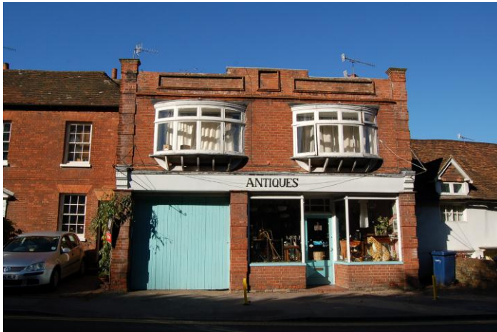
Figure 15: 72A Ockford Road
